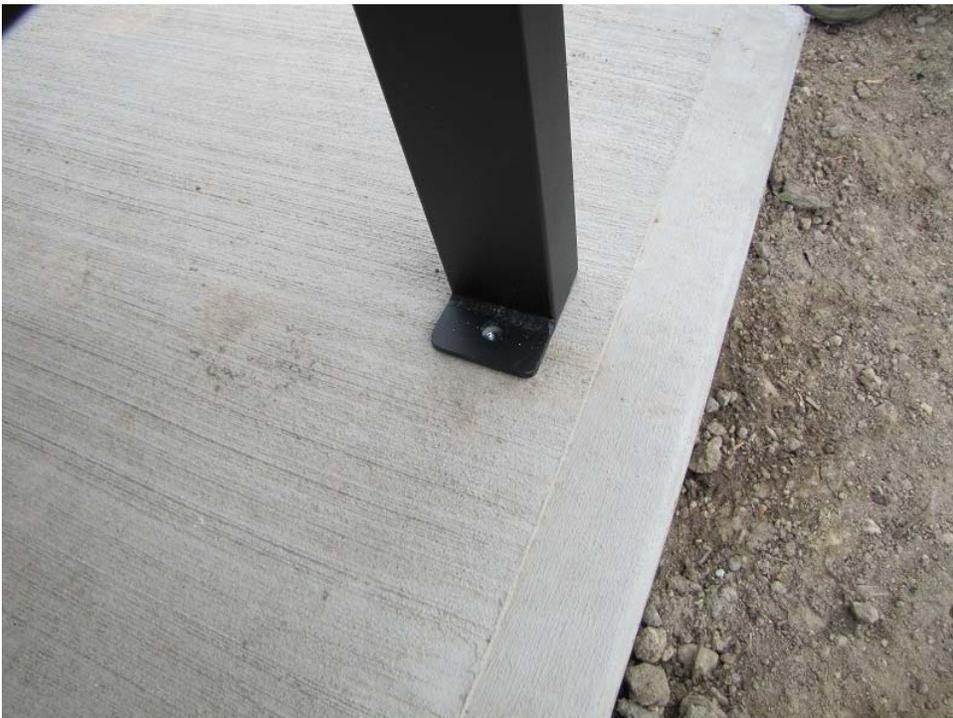
10. Secure bench to the anchor with bolt supplied.
