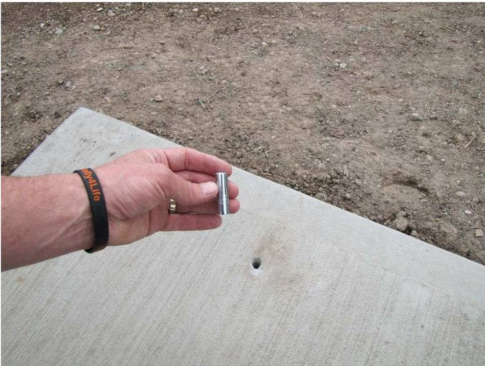
8. Hammer the anchor with the supplied post to expand the base securing it to the concrete.
