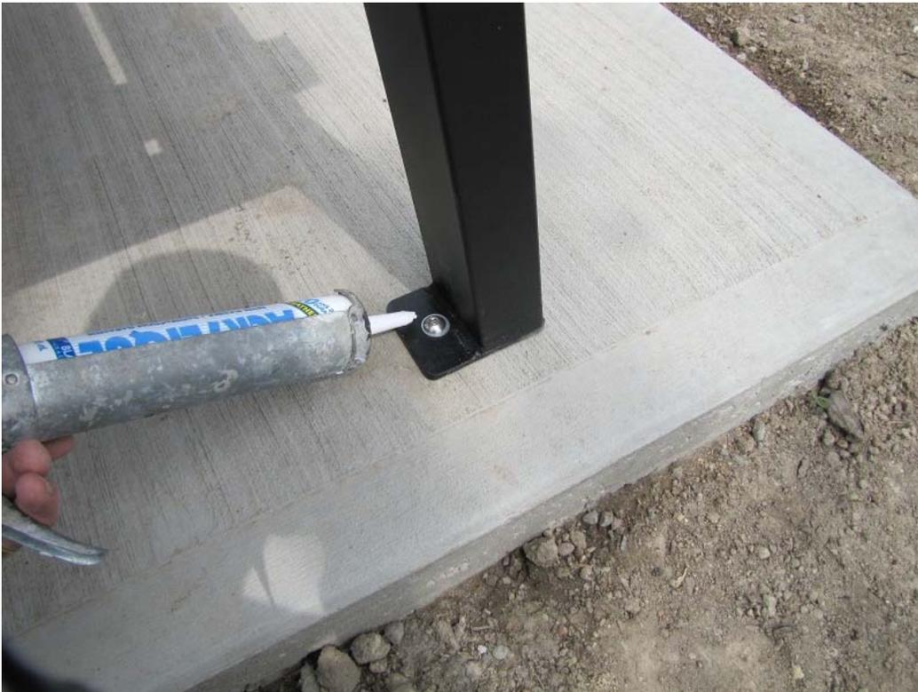
12. Paint the top of the fastener with a color to match the bench.
