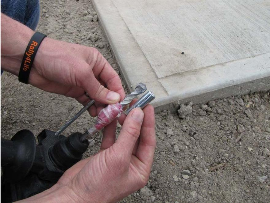
5. Drill the holes to a depth of 1-5/8" (as suggested by the anchor manufacturer).
