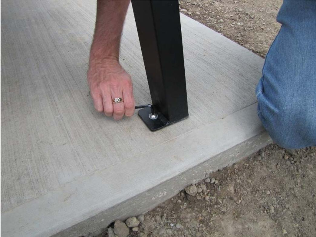
11. Fill the top of the fastener with silicone – this will deter vandalism or removal of the bench should someone have the appropriate tool,
