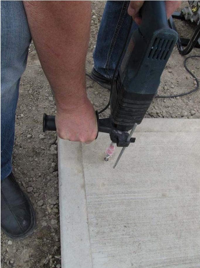
6. Blow out the holes to remove all the concrete dust and debris.
